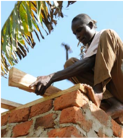
Building Eco-San latrines in Uganda.
