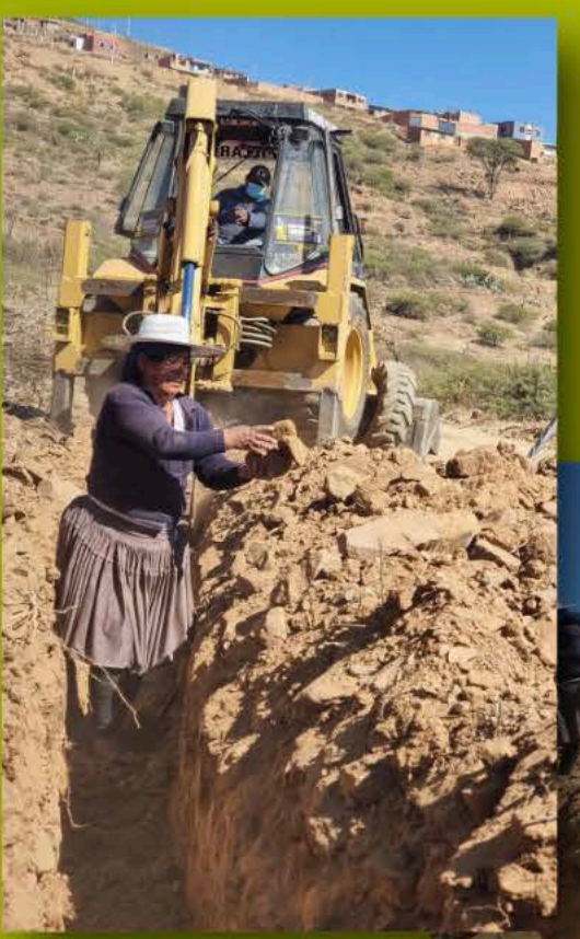
Women working on trenching for the water distribution system in Arbiesto (Cochabamba)
