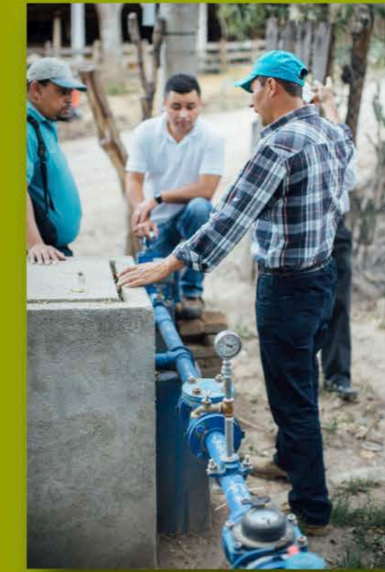
Community water system – water meter
