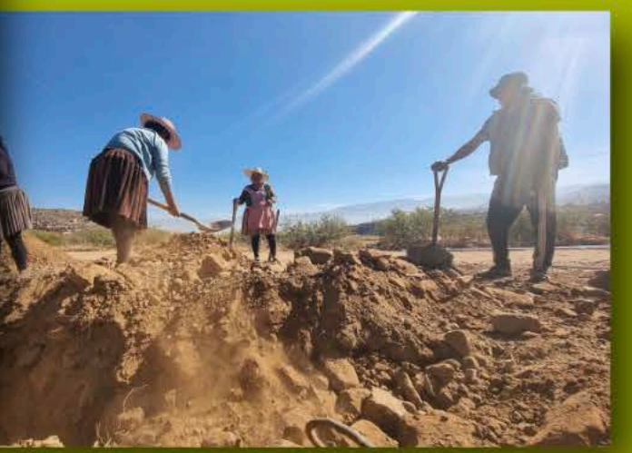
Women working on trenching for the water distribution system in Arbiesto (Cochabamba)
