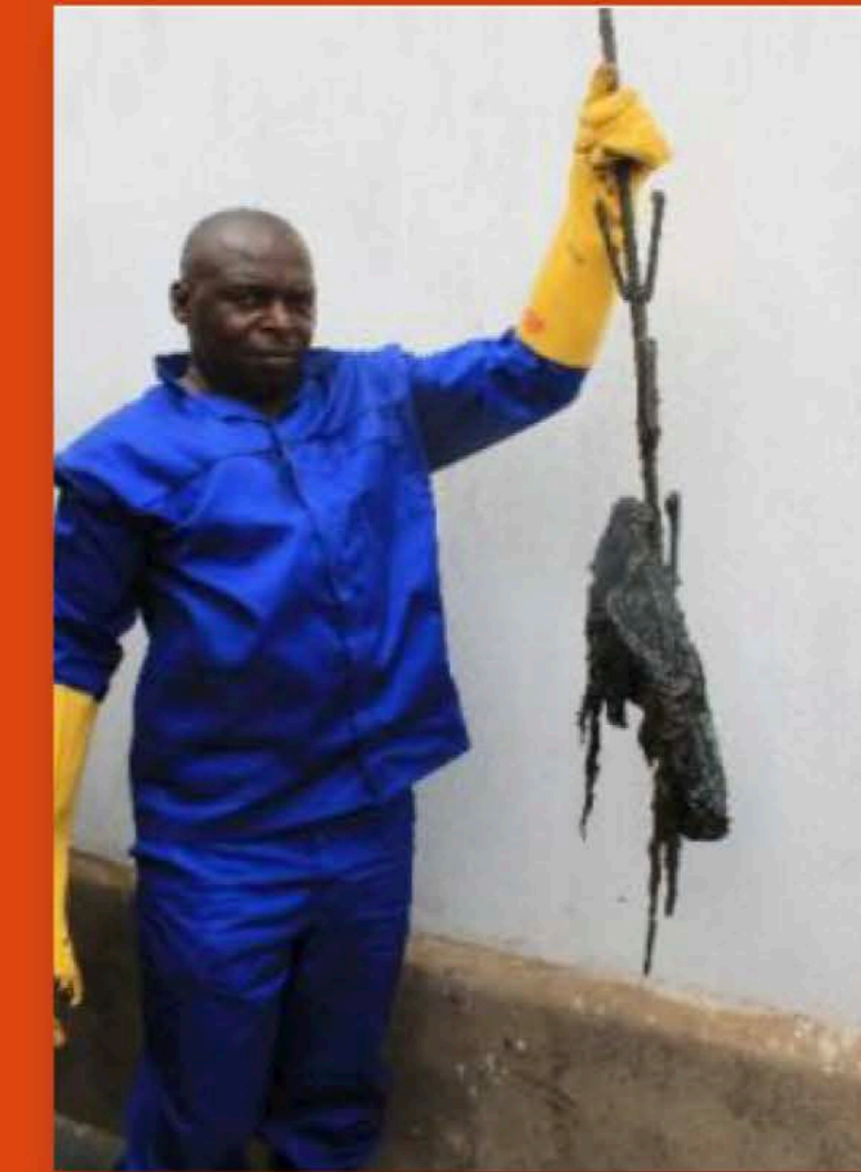
Pit emptier "fishing" garbage out of a latrine pit before emptying the fecal sludge -Photo courtesy of Steve Sugden
