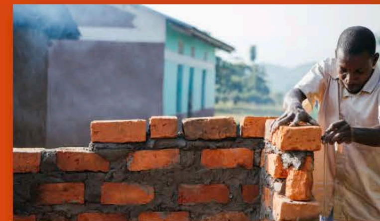
A mason constructing the walls of a school toilet facility
