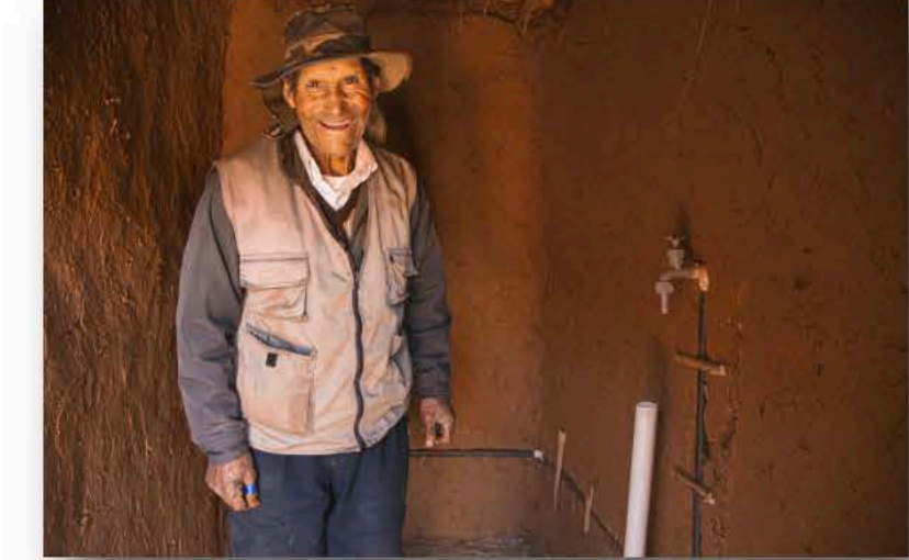
Guillermo building his new bathroom in Arani (Cochabamba)
