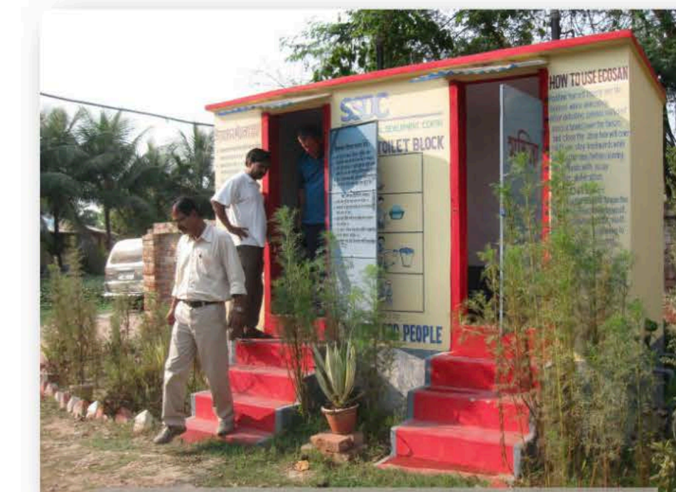
Community toilet (West Bengal) – Photo courtesy of Rajashi Mukherjee
