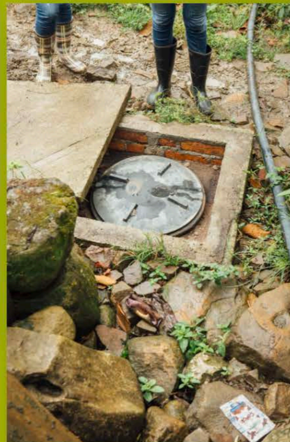
Household "biodigestor" (septic tank)
