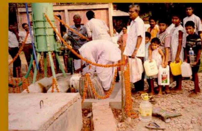
Arsenic filter near Maslandapur, North 24 Parganas (2003) – Photo courtesy of Arun Deb
