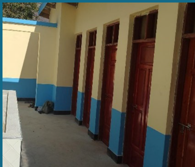
Installed hand washing station and inside look of girls latrine
