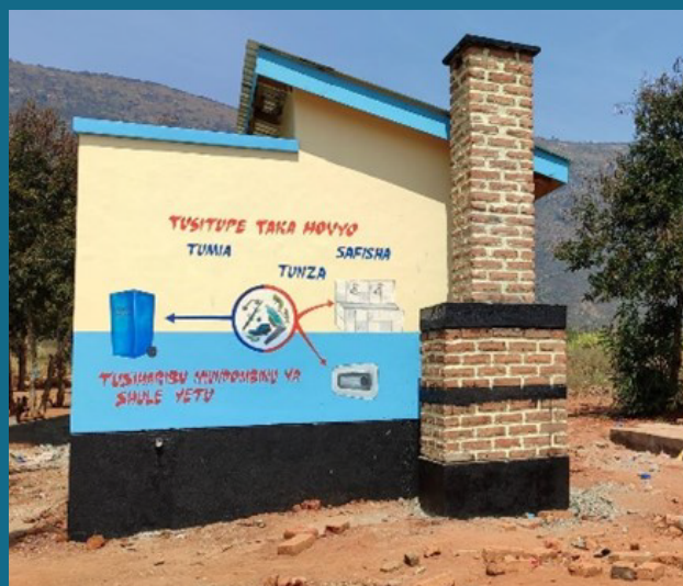
Special MHH room attached with Incinerator for Menstrual waste management
